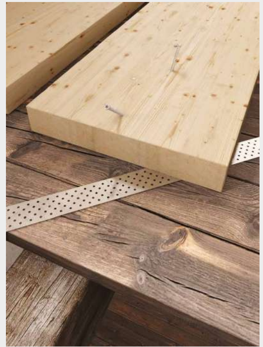
Restoration of existing timber floor using glulam beams and VGZ connectors.
